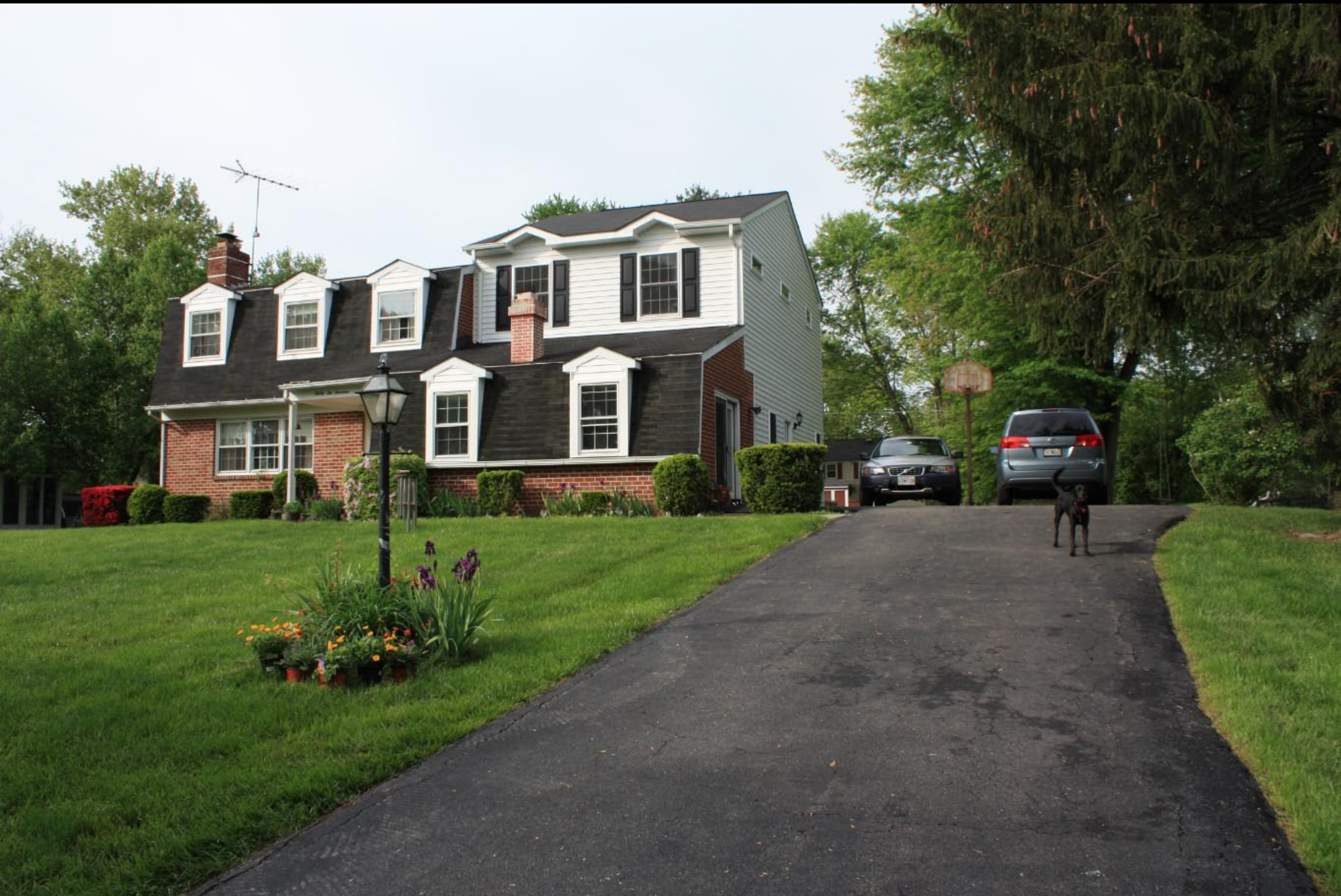
The additiion, on the right in white
